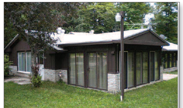
Surrounded by state land , perfect for conservationists and nature lovers. Three bedroom, 2 bath, nicely maintained, neat and clean cabin on approximately 5 acres, being sold with some furnishings. Outdoorsman's paradise. On a year-round county maintained road. Mixed trees abound, giving shelter to native wildlife. 428304 $89,500
