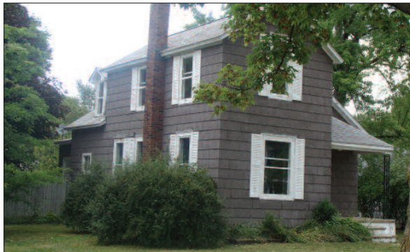
Great 3 bedroom in-town Boyne City home - one of those older houses with original hardwood floors and interior woodwork, great staircase and wonderfully decorative windows. Large detached garage will be invaluable if you plan on DIY refurbishing. Really ideal family location, close to town, shopping, schools and churches, or could be a delightful second home. 431102 $74,900
